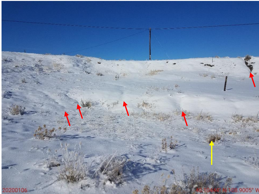
Photo 1: Photo taken from the south end of the Location, facing north. Photo shows overview of the Location and well marker. Photo shows an open pit on the south end of the location (yellow arrow) and the well marker. Photo also stormwater erosion degradation on Location (red arrow).
