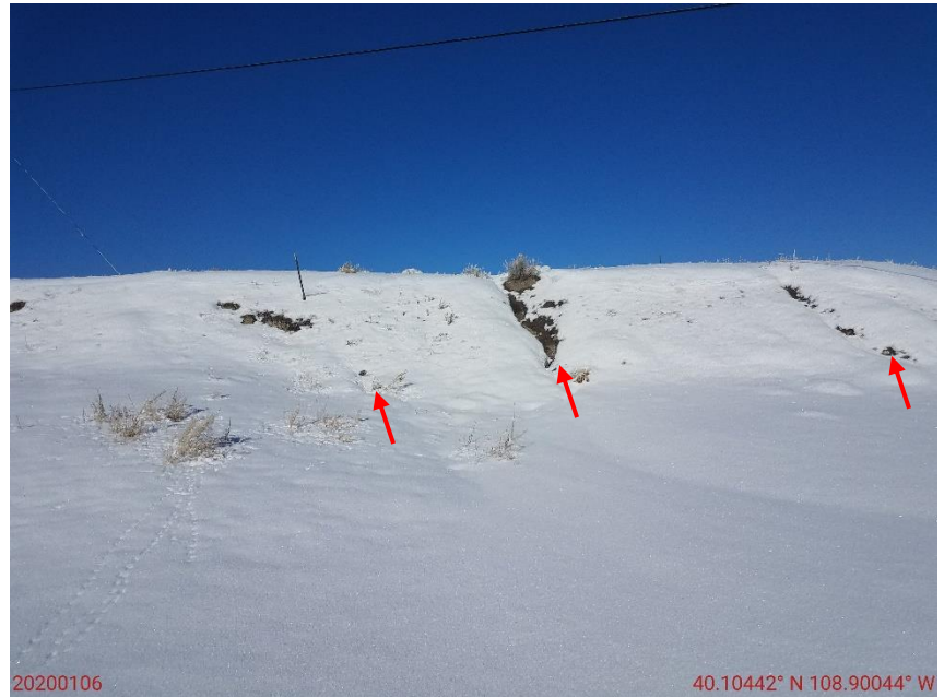
Photo 4: Photo taken from the north end of the Location. Photo shows erosion degradation observed on the cut slopes.
