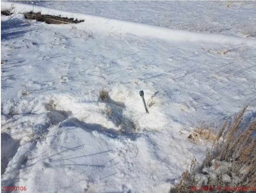
Photo 3: Continued from photo 2: Photo shows anchor associated with the utility pole left on location.
