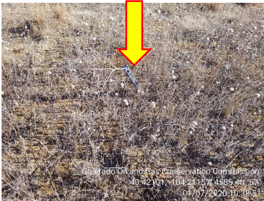
Photo 3 – SE Deadman/Guy line anchor – Not Marked
