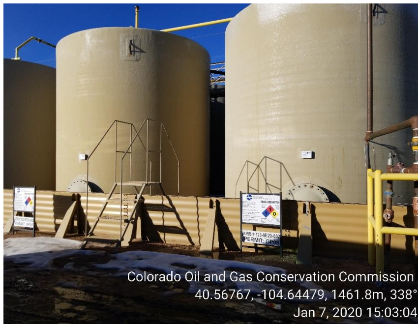
Photo 3: No BBLS labeling on H2O tanks
