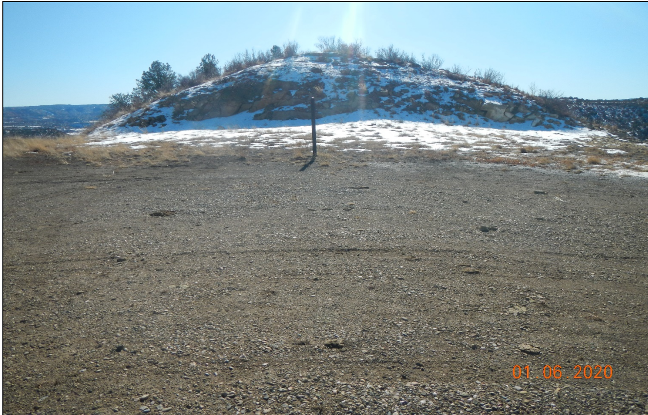
Photo 4. The equipment has been removed from the location and a permanent well marker is installed.
