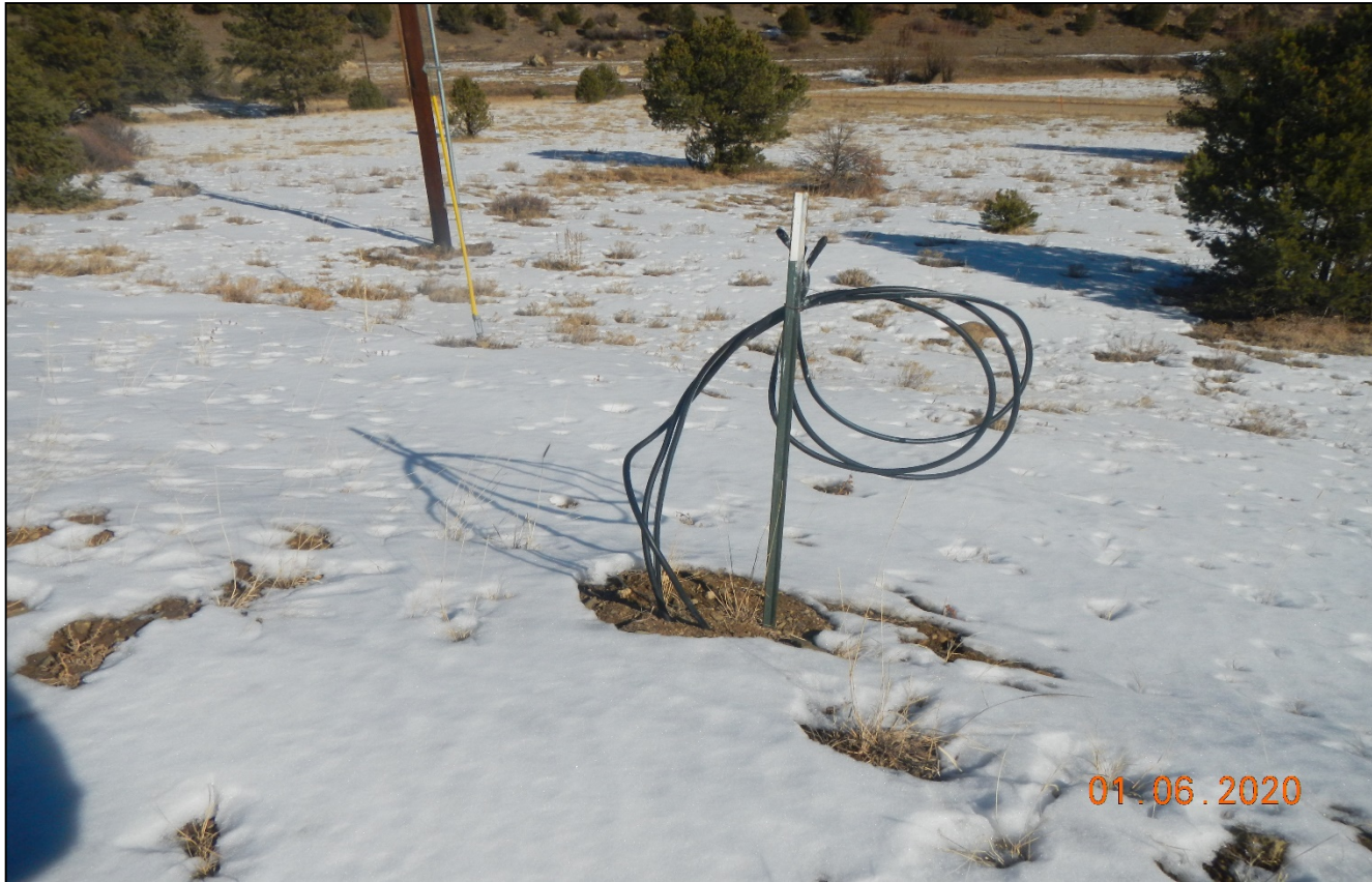
Photo 4. The powerline cable has not been removed. The wires are unsecured which is a safety concern
