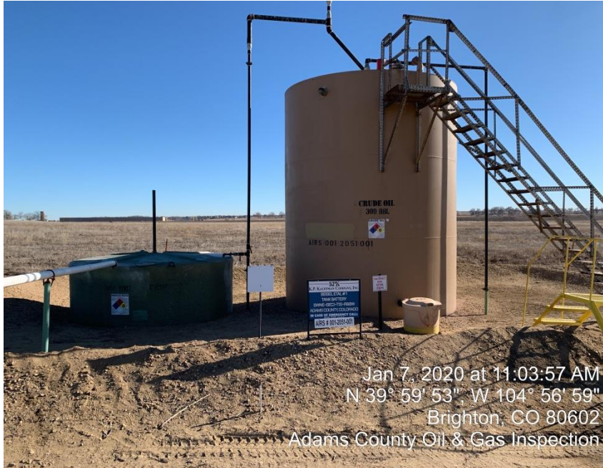
Photo#1 Production tank and Produced Water Tank
