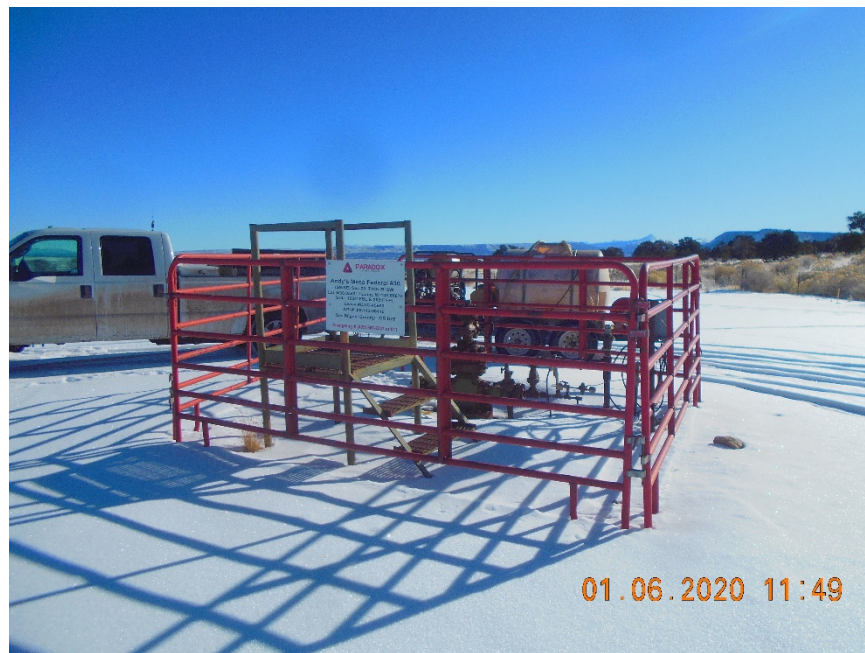
Temporarily Abandoned Wellhead with fence.
