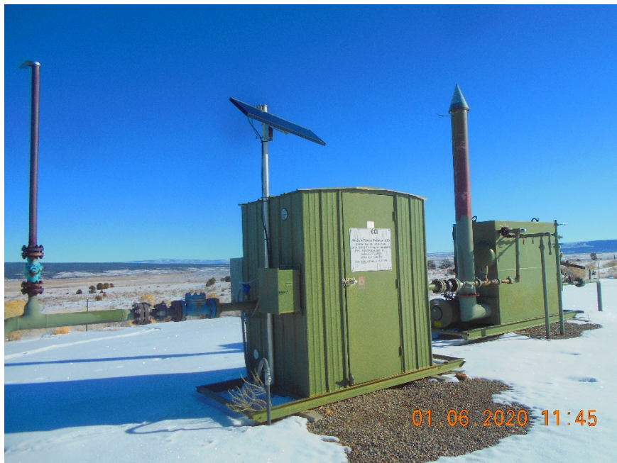
Separator and Meter housing with sign
