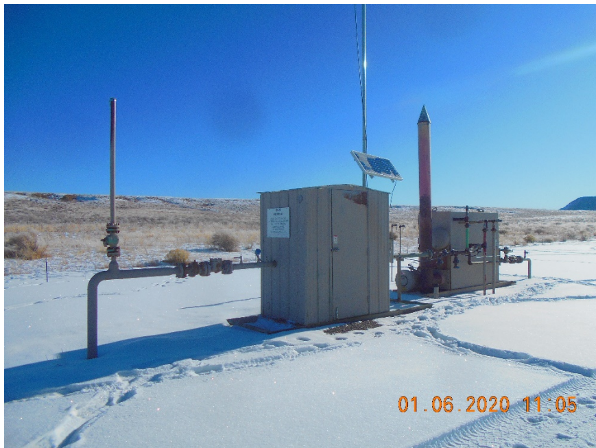
Separator and Meter housing with sign
