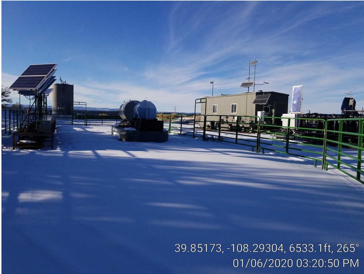
Photo 1. Battery & separator.
