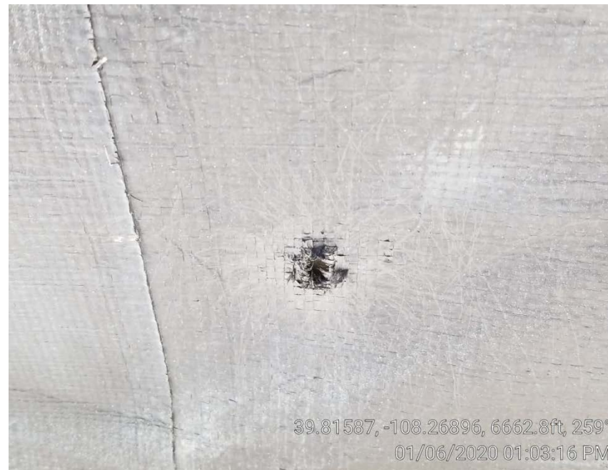
Photo 6. Tank secondary containment liner hole.
