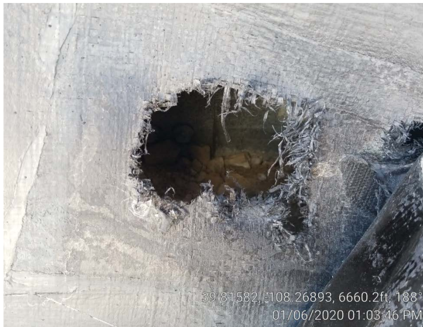
Photo 5. Tank secondary containment liner hole.
