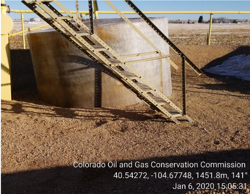
Photo 3: Base of berm repaired
