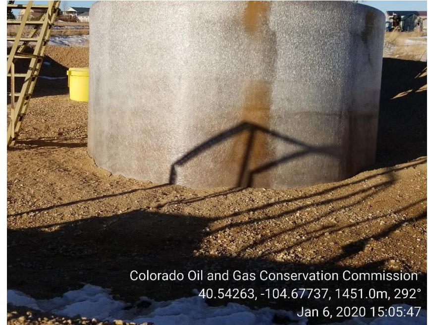
Photo 4: Base of berm repaired
