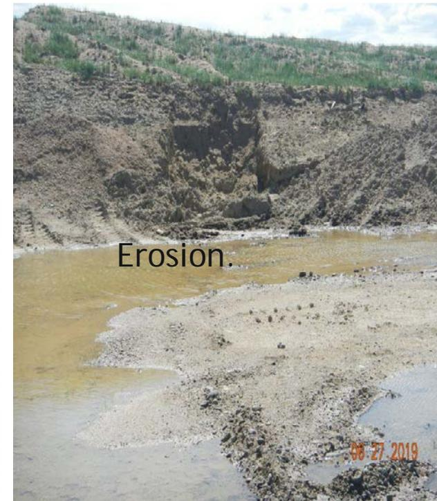
1002. c. - Protection of soils Mutual LOC# 324757 -Topsoil was not protected from wind and water erosion, and weed establishment
