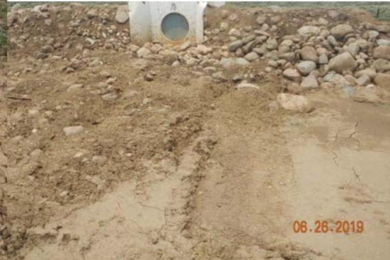
French Drain: Inadequate or improper installation of BMP.
