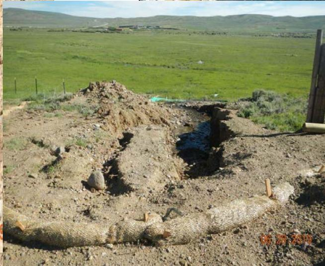
Silt Fence installation: *Inadequate or improper installation of BMPs.*
