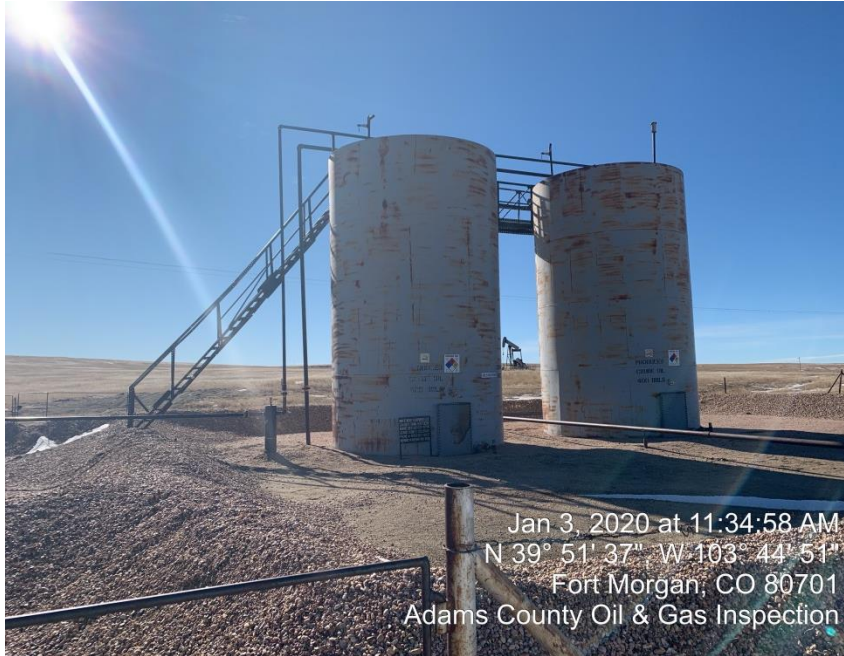
Photo#1 Production Tank/Tanks need painted
