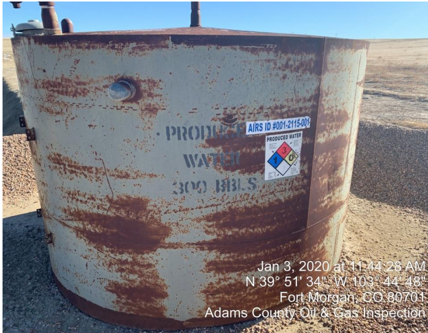
Photo#5 Produced Water Tank/ Tank needs painted
