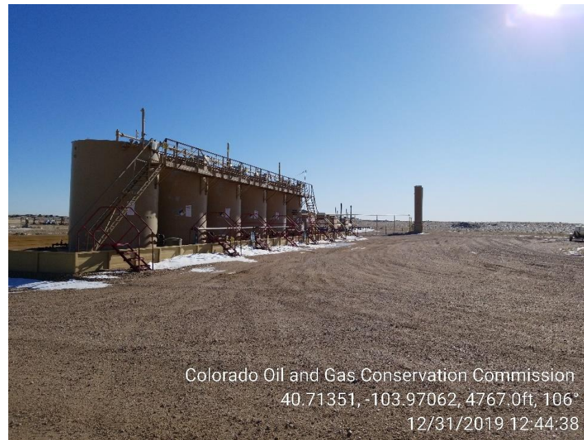
Photo 2 – Tank Battery
