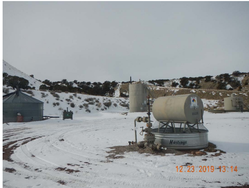
Photo 1. Overview of location taken facing west.
