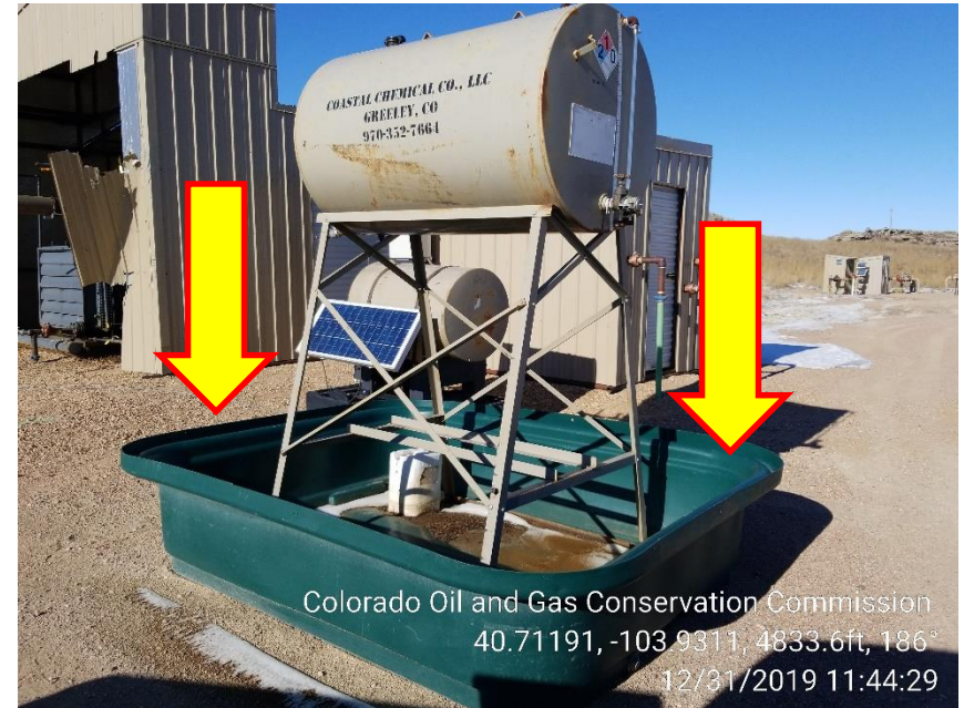
Photo 4 – No Wildlife netting on Secondary Containment
