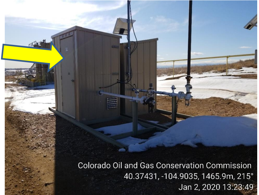
Photo 6: Disconnected gas meter
