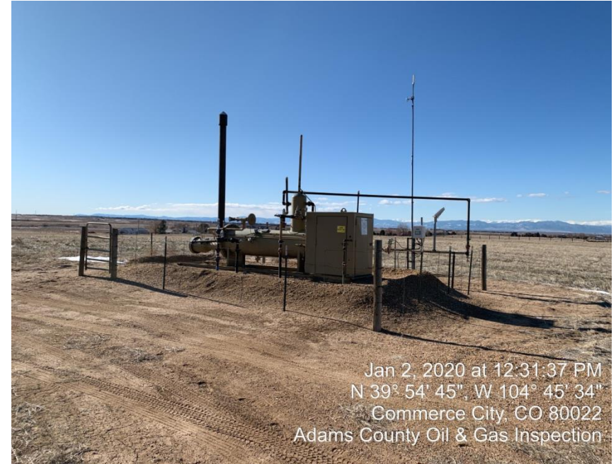
Photo#2 Separator/Gas Meter/RTU
