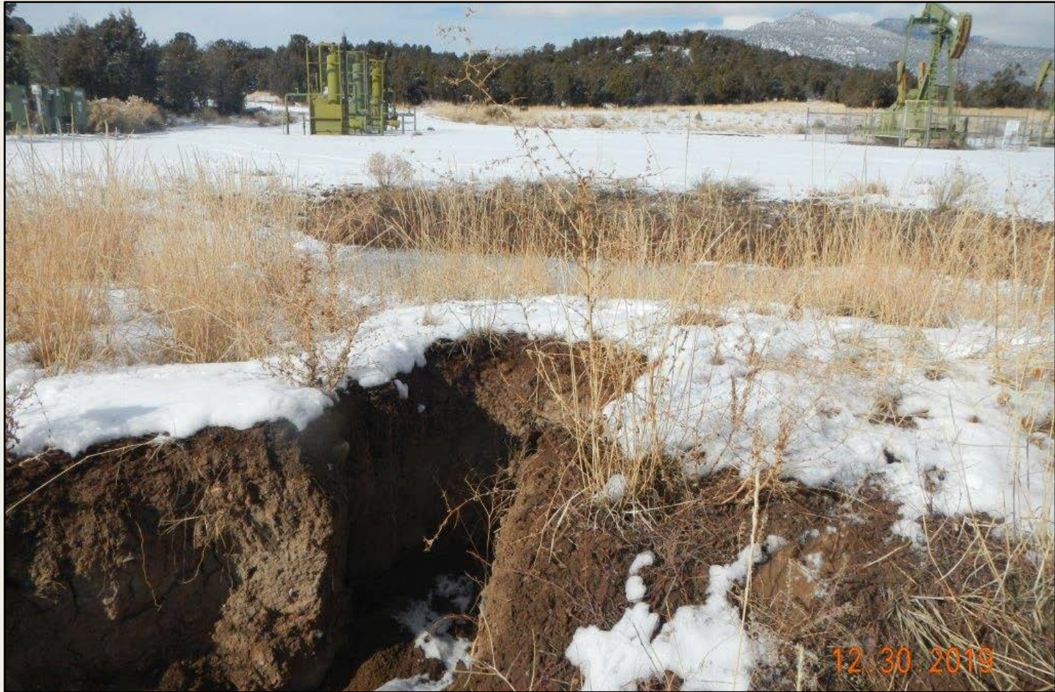
Photo 3. View of erosional channel where the southern sediment trap is breeched. This sediment trap does not have a stabilized overflow outlet.
