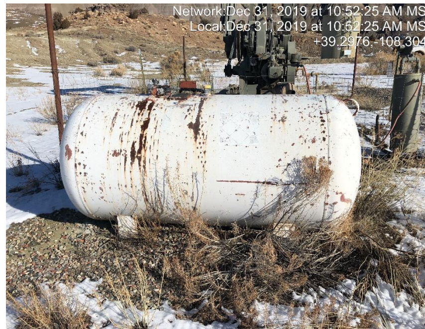
Photo #0333 tank by wellhead is not properly labeled.
