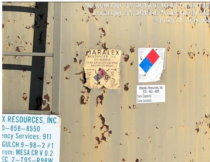
Photo #0329 Tank label and placards are weathered and not legible.
