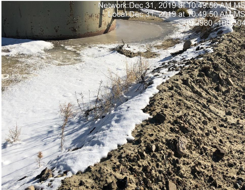
Photo #0330 weeds inside tank containment
