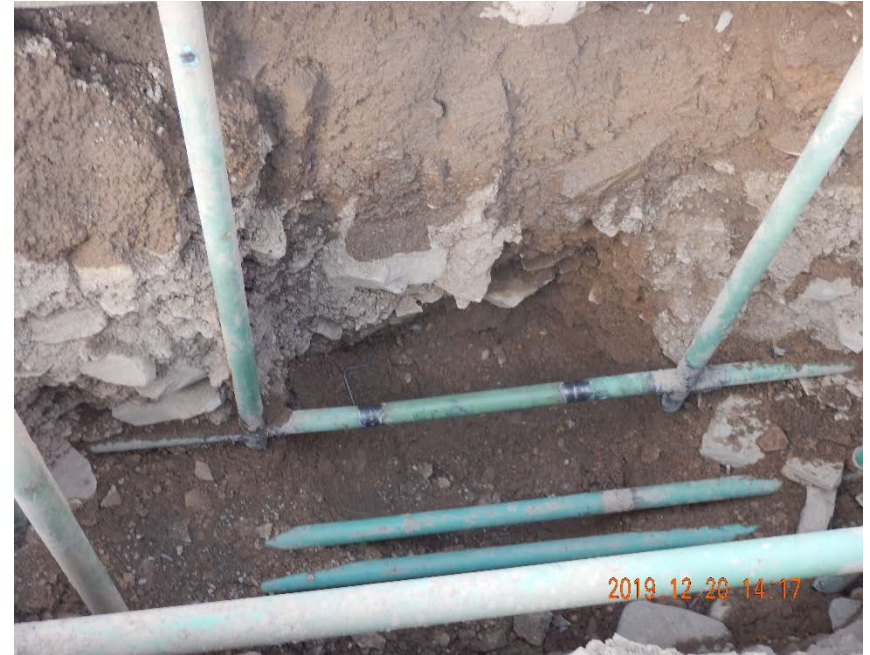
Photo #10 – View of repaired dumphine inside of excavation.
