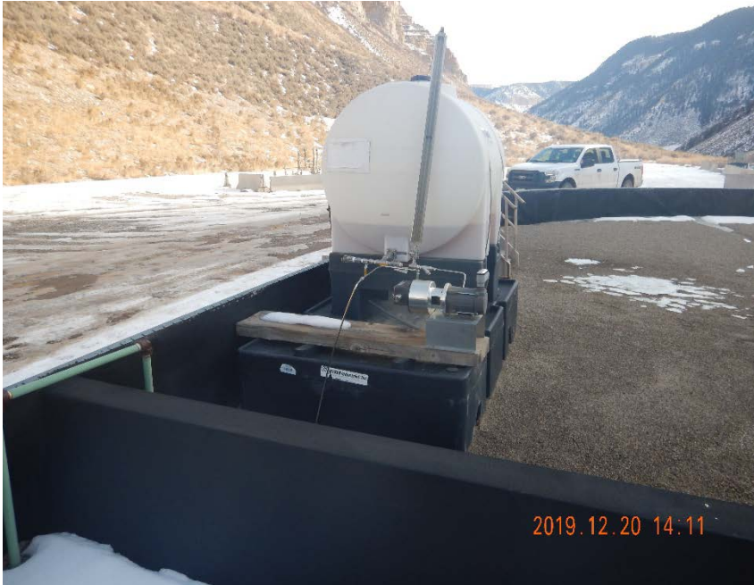
Photo #9 – Day tank inside of secondary containment.
