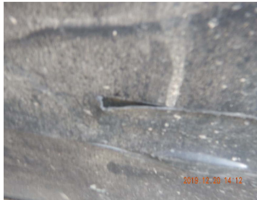
Photo #6 – Damaged section of tank battery liner, near tank battery loadout (1).
