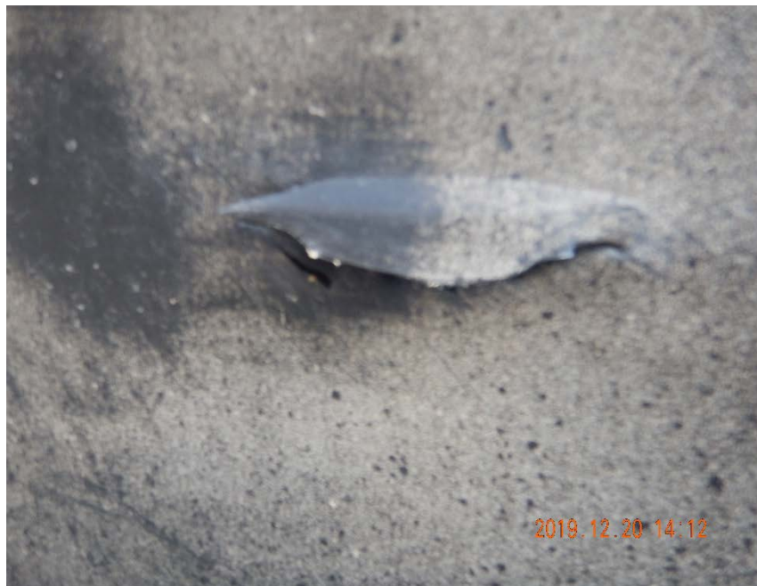
Photo #7 - Damaged section of tank battery liner, near tank battery loadout (2).
