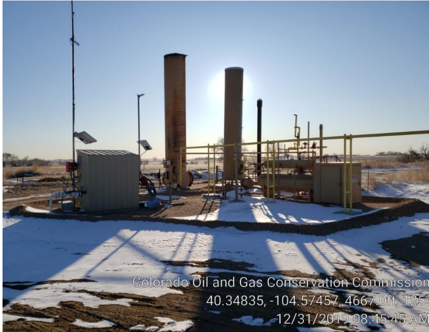
Photo #3 Separator, ECD's & Meter Run
