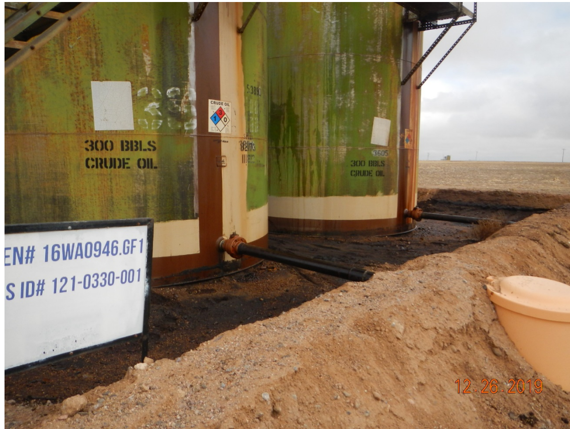
Photo # 2 – South side of tank battery oil stained soil in berm
