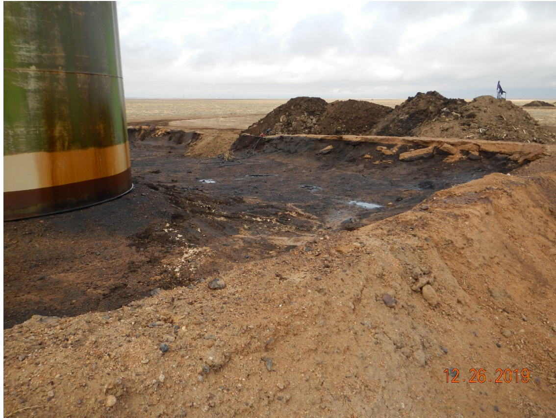
Photo # 3 – Northeast corner of tank battery, oil stained soil in berm, oily soil stockpile north of battery berm
