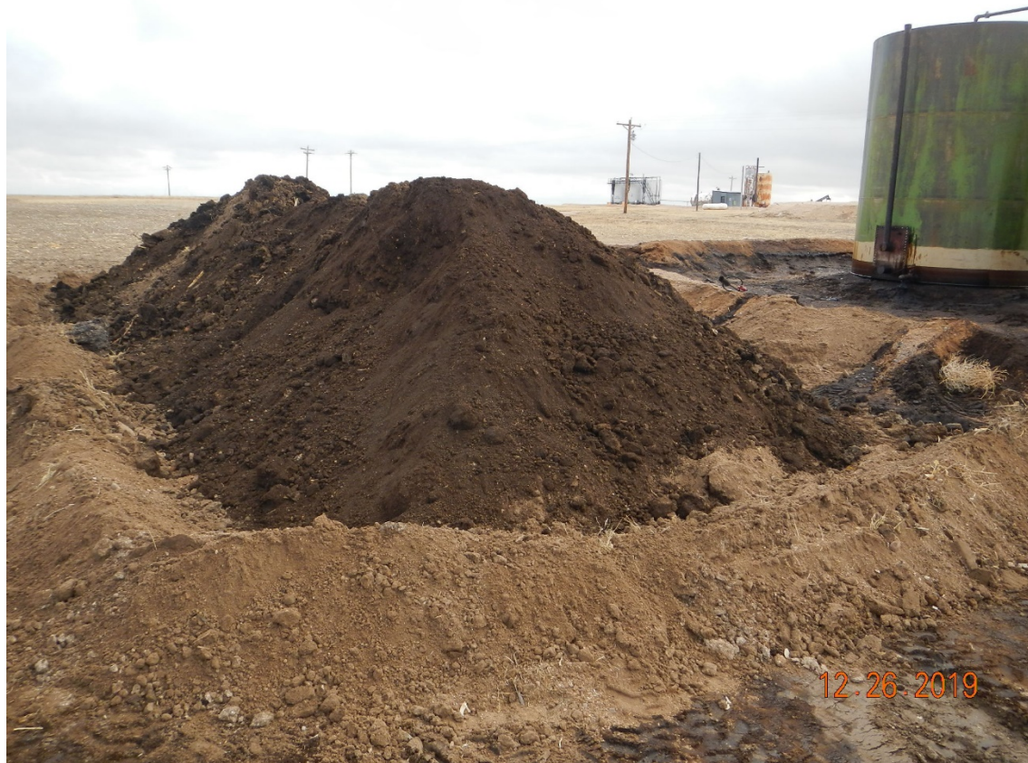
Photo # 4 – Oily soil stockpile north of battery berm
