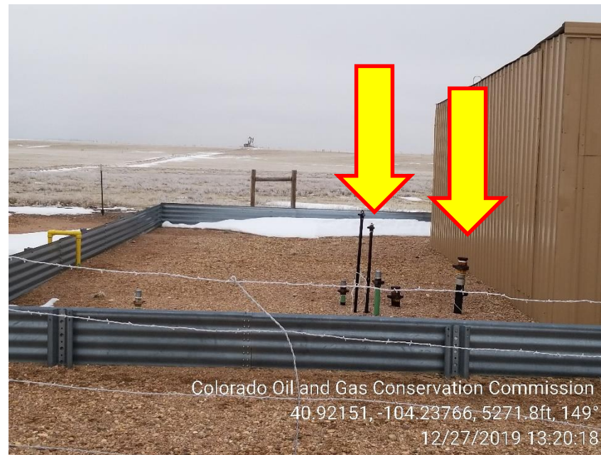
Photo 2 – Unmarked Risers
