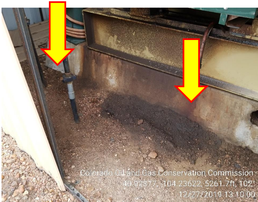
Photo 3 – Stained Soil at gas engine
