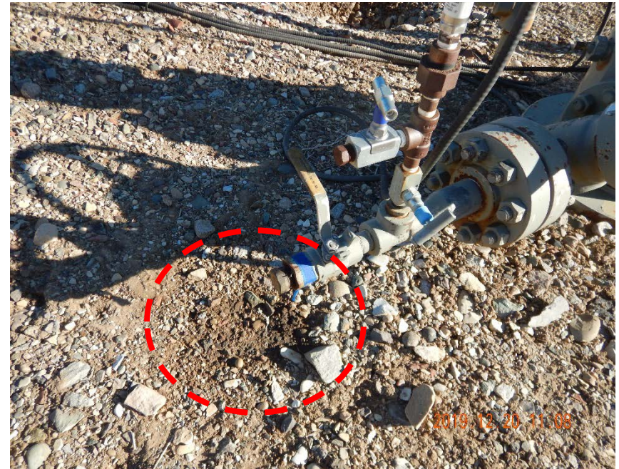
Photo #10 – Localized accumulation of oil-stained soil observed on north side of PB15 Clem Jr. 15-6 wellhead.
