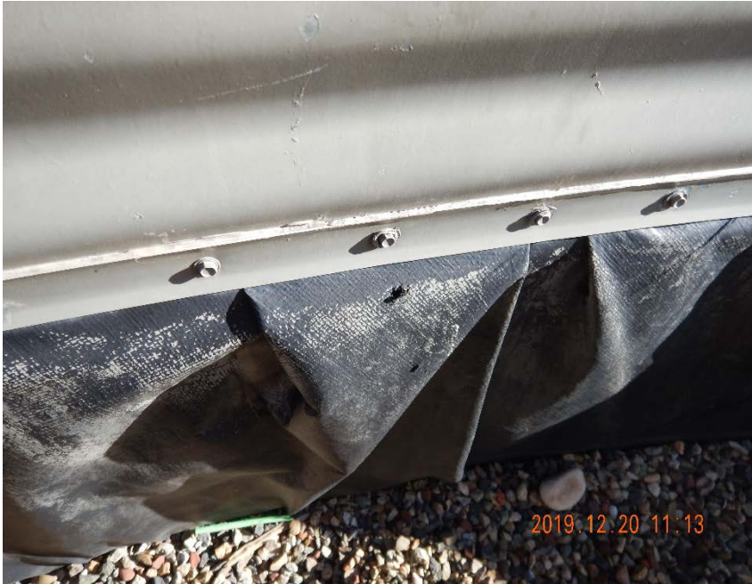
Photo #7 – Pinhole observed in liner inside of tank battery secondary containment area.
