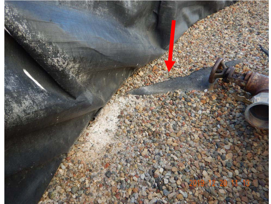
Photo #8 – Ends of liner panels were observed sticking up from bottom of containment area on inspection date.
