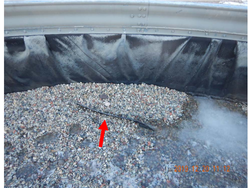
Photo #6 – Tank battery secondary containment area contained ice and fluid on inspection date. No hydrocarbon sheens or odors were observed inside of secondary containment area on inspection date.
