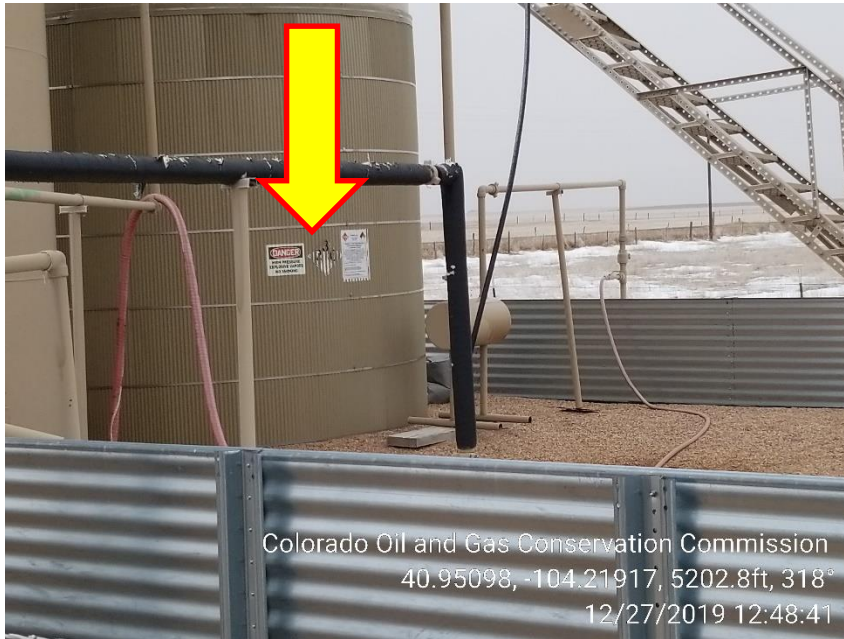
Photo 3 – NFPA Label on Produced Water tank is fading, missing capacity label.
