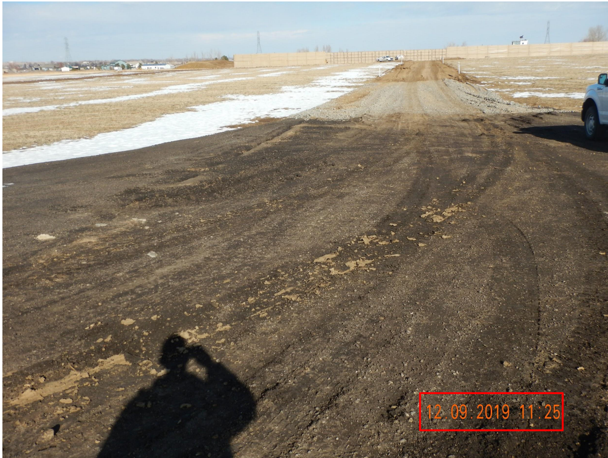
Photo 1. Photo taken from the entrance of the location on 12/9/2019, facing North. The current vehicle tracking device BMPs are not adequate to be in compliance with Rule 1002.f.(2)F.
