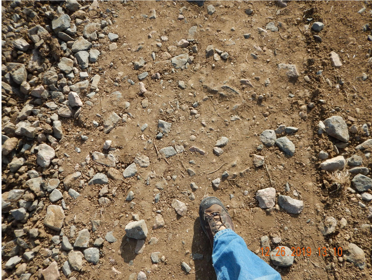
Photo 4. Close up photo taken from a portion of the rip-rap BMP that is not in proper functioning condition.
