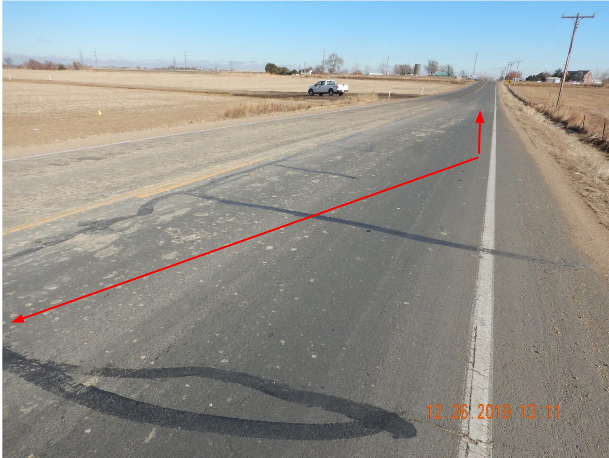
Photo 5. Photo taken west of the entrance on CR 2, facing East. Photo illustrates material tracked onto the county road.
