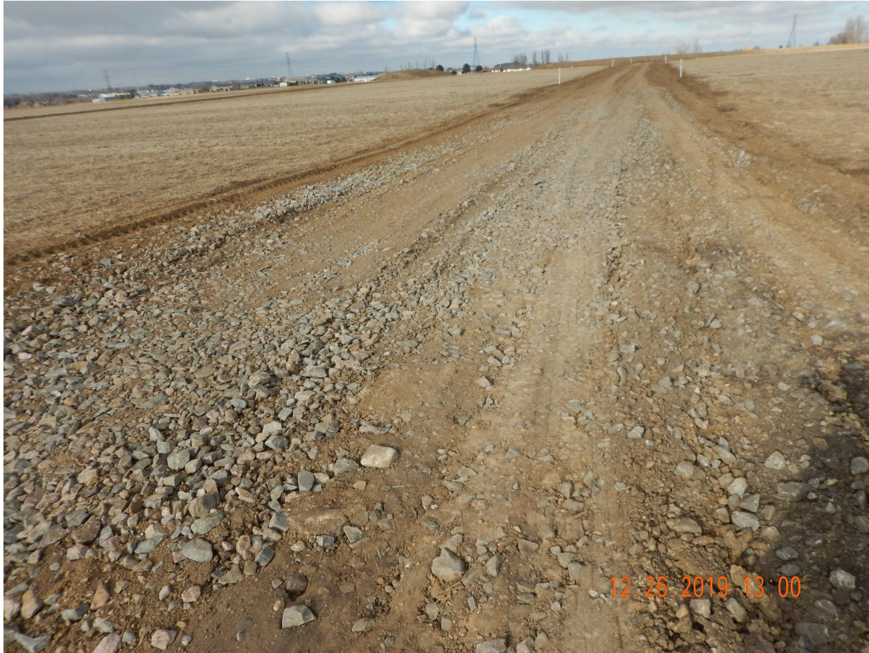
Photo 3. Photo taken from a portion of the vehicle tracking device BMP, facing North. The current vehicle tracking device BMPs are not adequate BMPs for this location.
