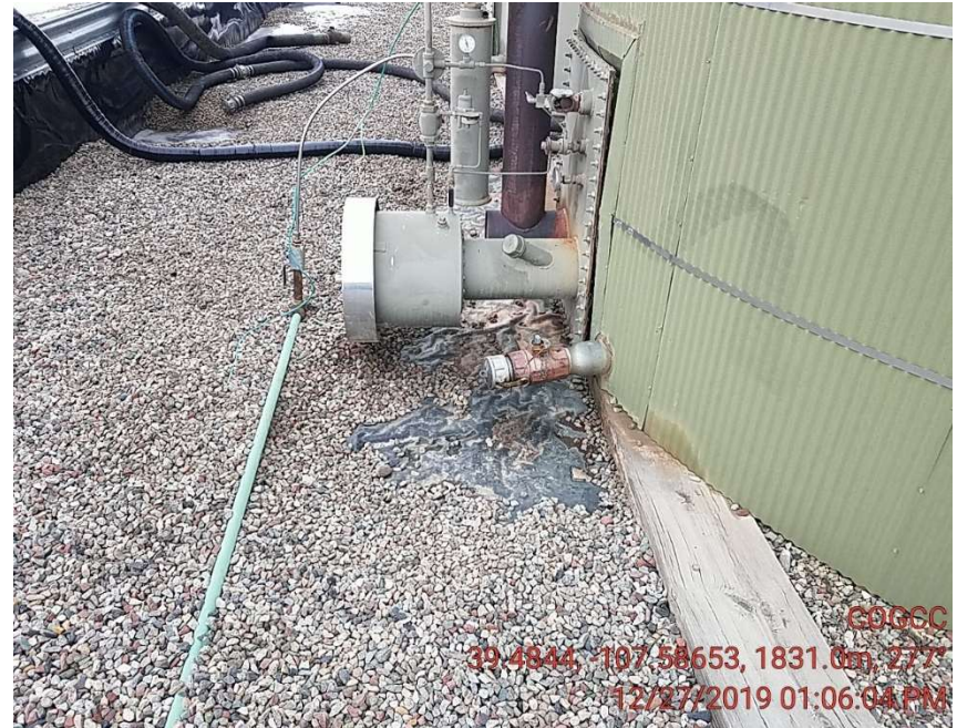
STAINED GRAVEL HAS BEEN REMOVED
