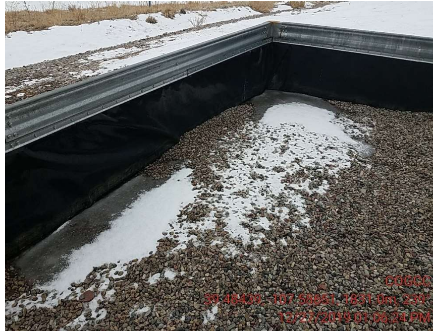
STAINED GRAVEL HAS BEEN REMOVED
