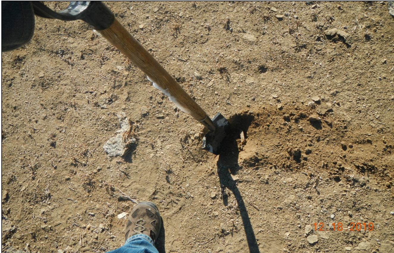
Photo 8. Soils seem compacted in areas. Soils need to be evaluated for proper decompaction.
