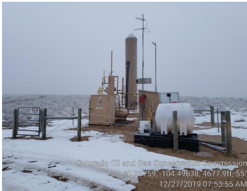
Photo #3 Separator, ECD & Meter Run.
