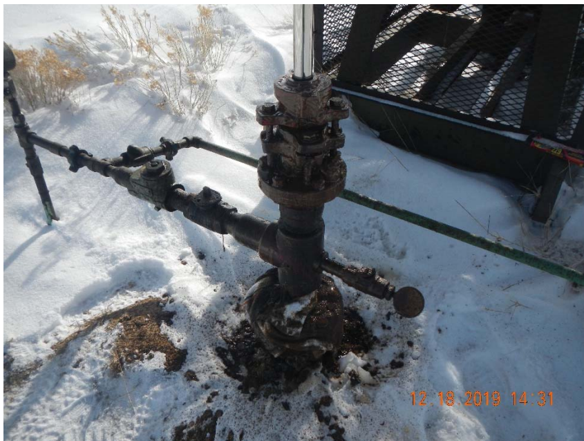
Photo 3. Close-up of wellhead with rags stuffed into it.
