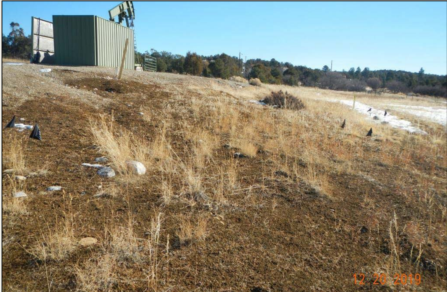
Photo 2. View of the southern fill slope from the southwestern corner facing eastward. Revegetation is progressing with grasses such as smooth brome, intermediate wheatgrass, and crested wheatgrass.
