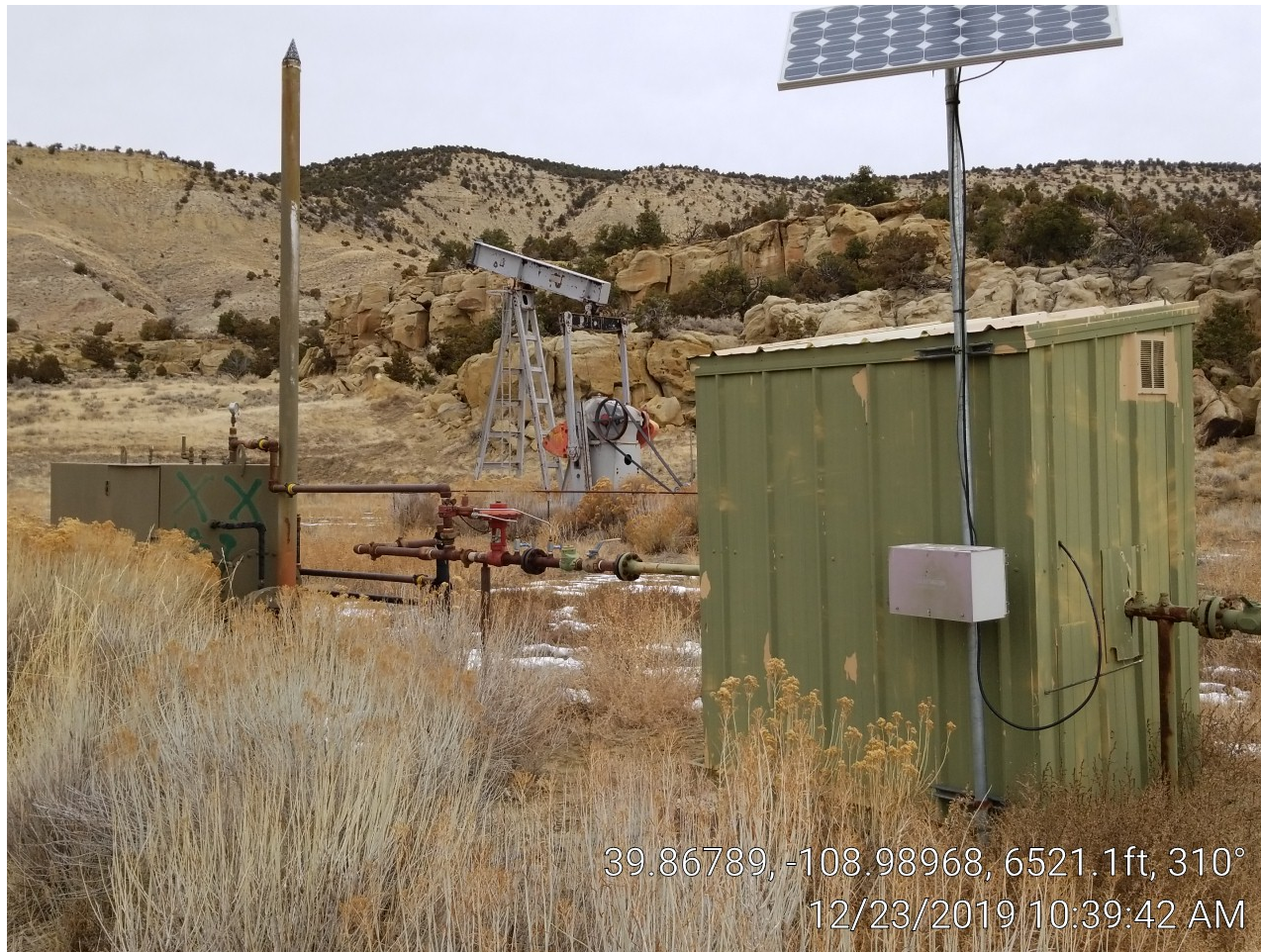
Photo 3. Meter building & separator.
