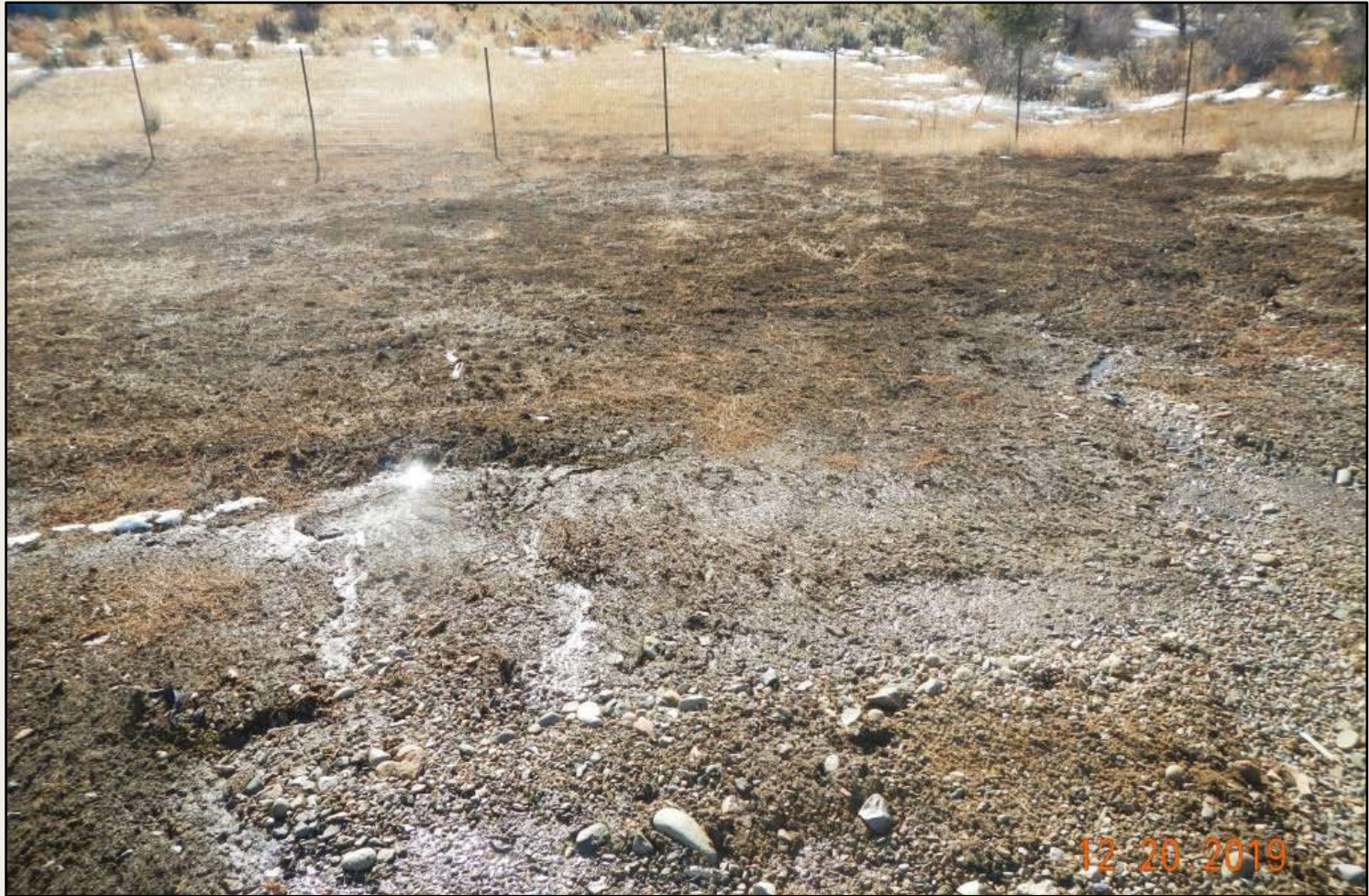
Photo 3. View of stormwater flowing downslope away from the well pad toward a drainage. No stormwater controls are in place.
