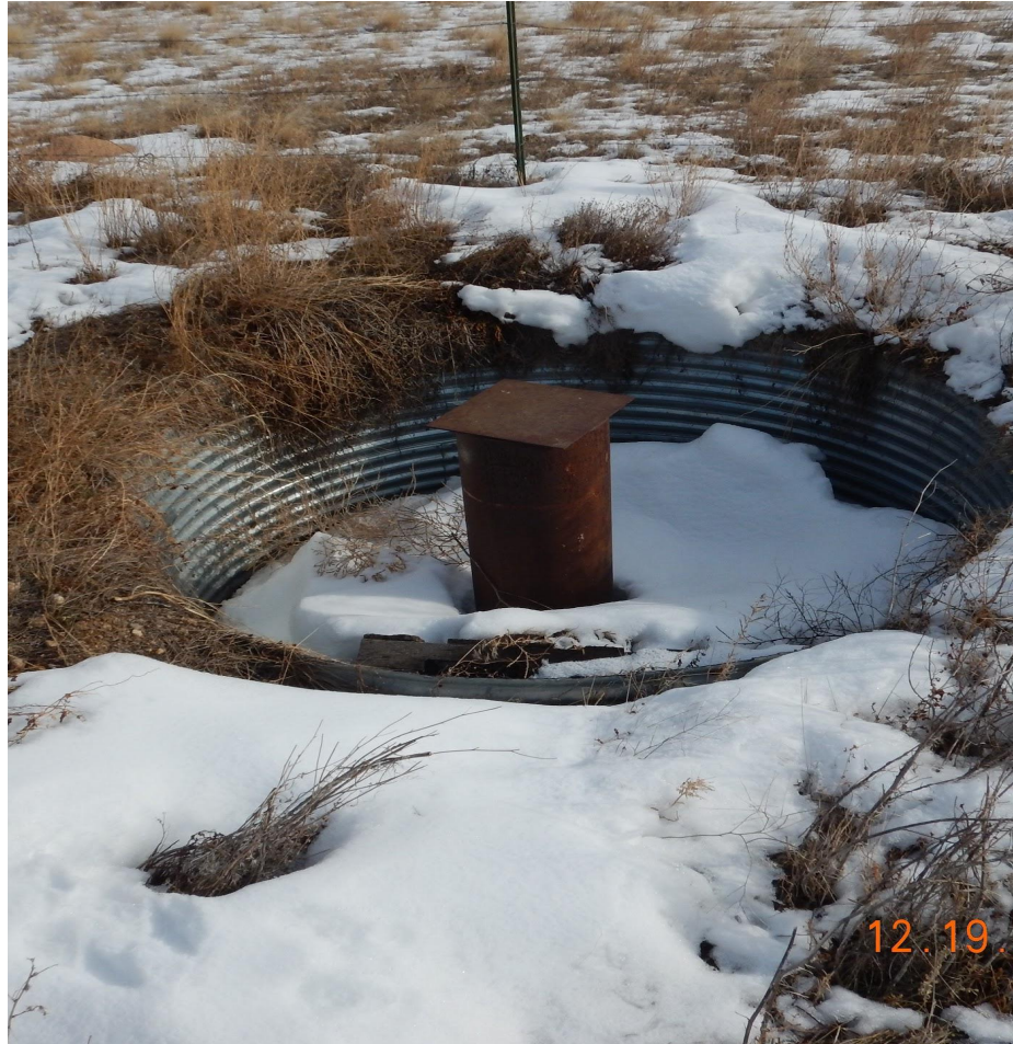
Photo 2. Close up photo taken from the well left with surface casing.
