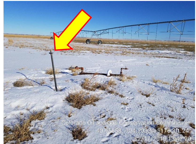
Photo 2 – Unmarked Riser at Wellhead
