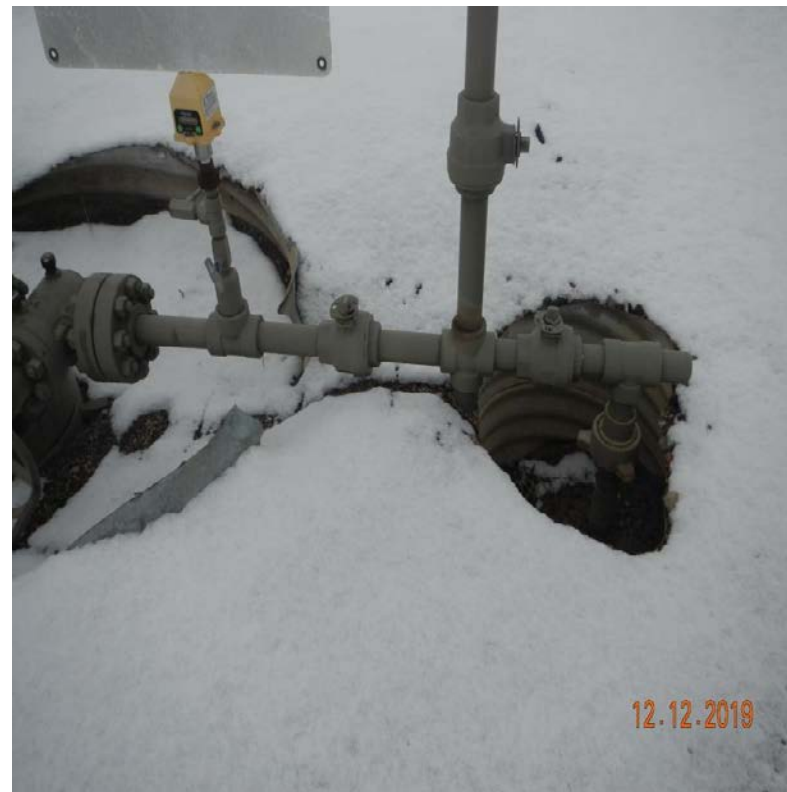
Photo#3: Small cellars (housing lines/valves) adjacent to Main well cellars.
