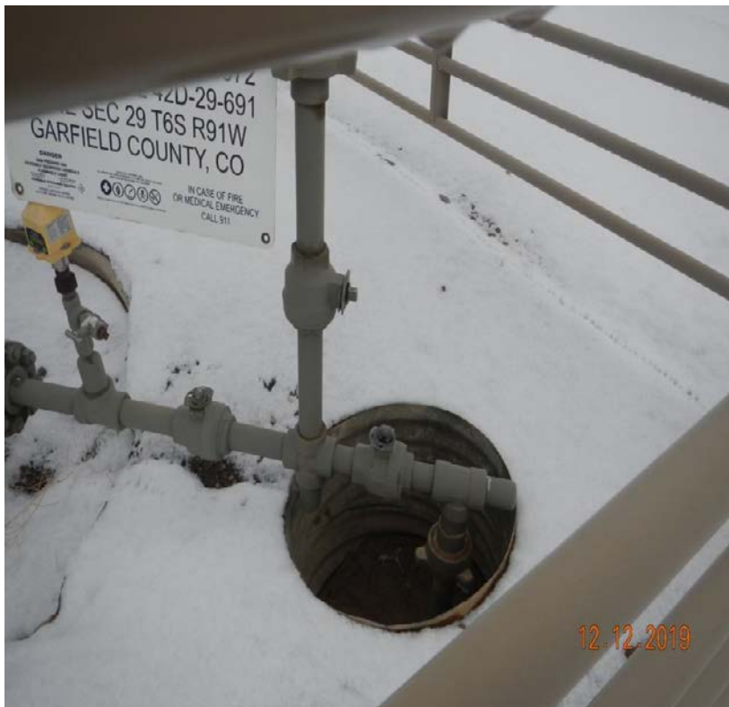
Photo#2: Small cellars (housing lines/valves) adjacent to Main well cellars.
