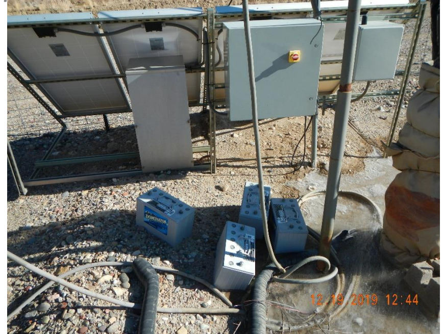
4 - batteries not properly stored sitting at injection well.
