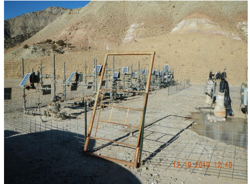
Gates on well head fencing are leaning
