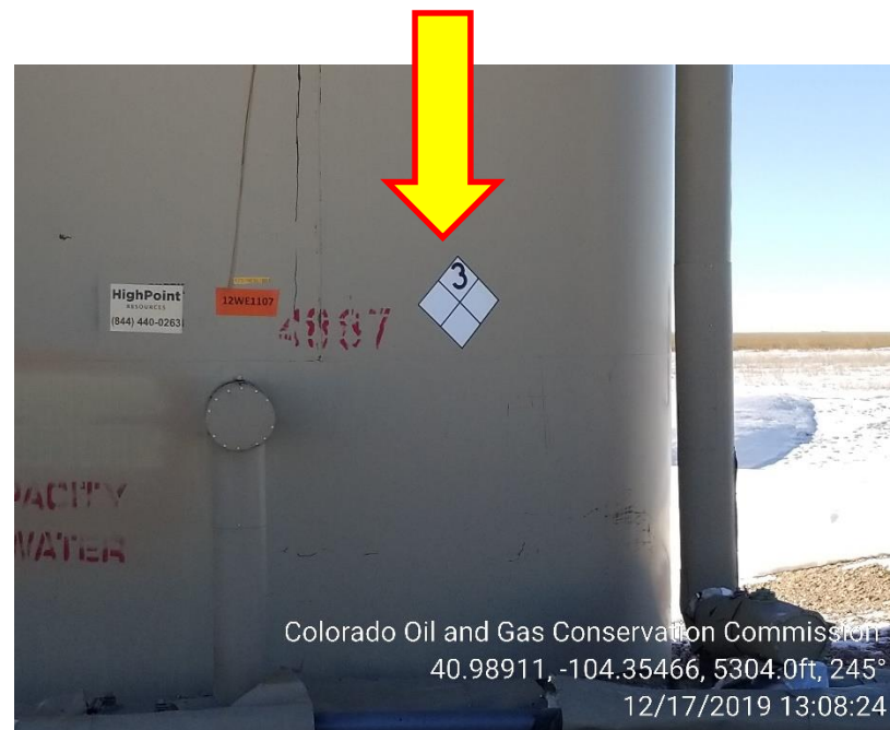
Photo 4 – North Tank – NFPA label has faded
