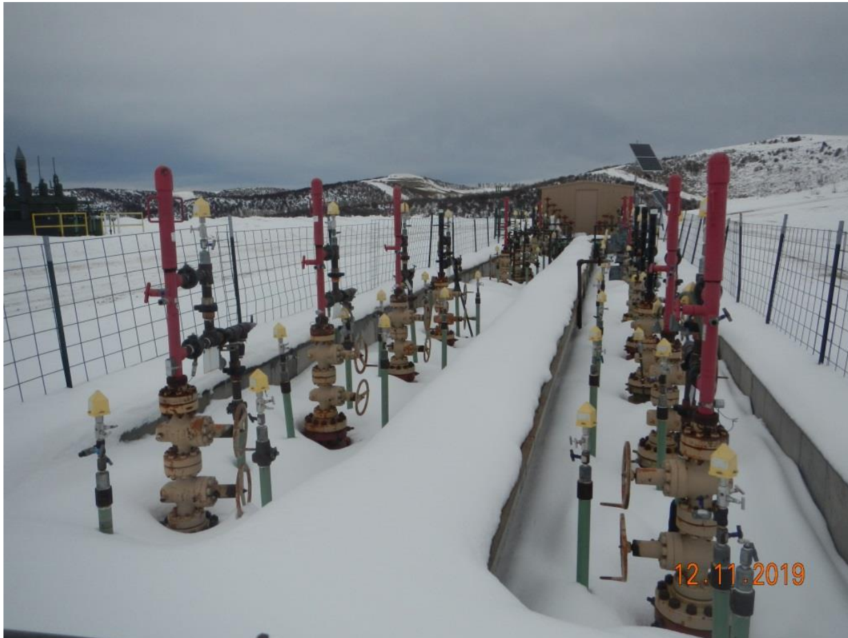
Photo#2: Overview of Well lineup and concrete cells.
