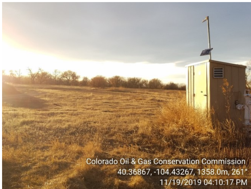
Photo #1 DOW 43-28 Battery site Abandoned | Most equipment removed Reclamation progressing Unused Gas meter run prior insp.
