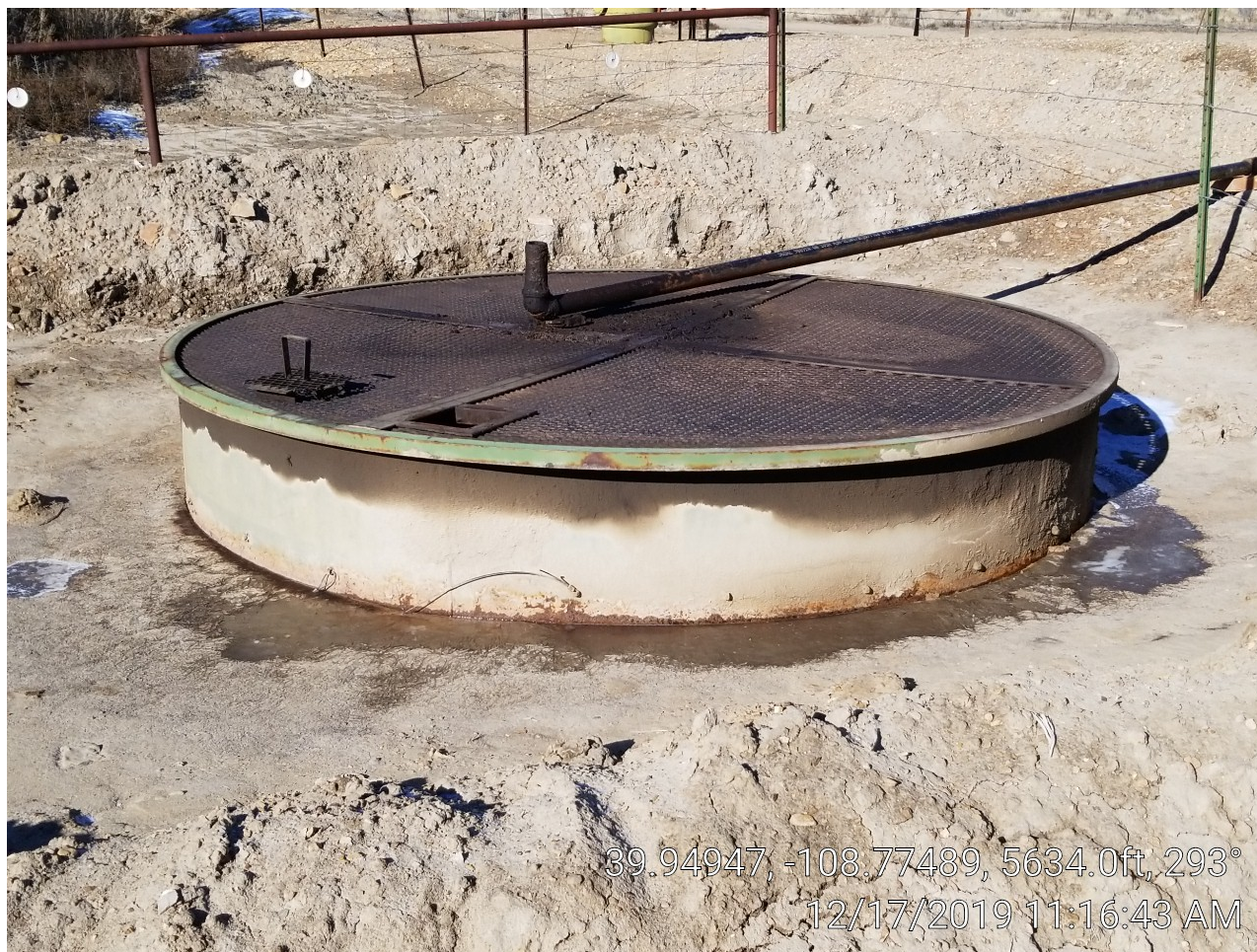
Photo 4. Partially buried tank.
