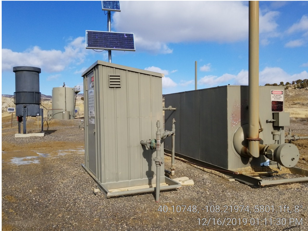
Photo 4. Combustor, meter building, and separator.
