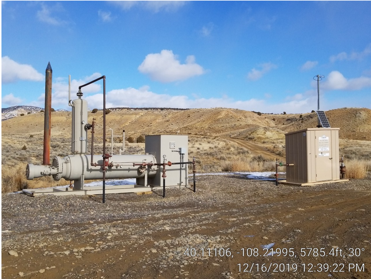
Photo 3. Separator and meter building.
