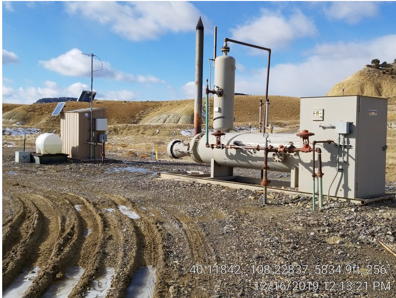
Photo 3. Meter building & separator.
