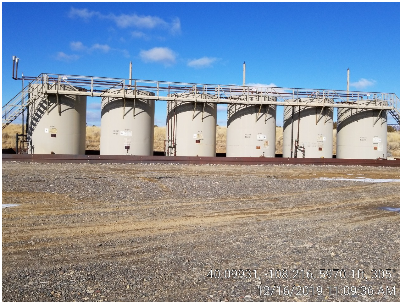
Photo 3. Tank battery.
