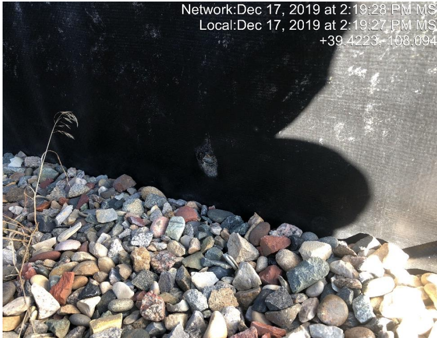
Photo #0275 Multiple holes in tank containment liner.
