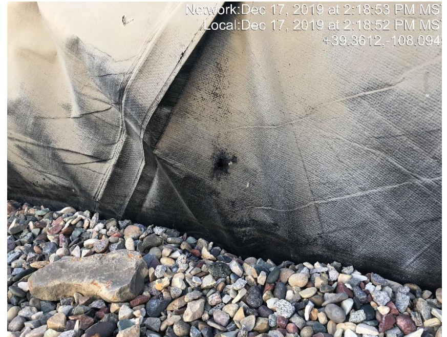
Photo #0274 Multiple holes in tank containment liner.
