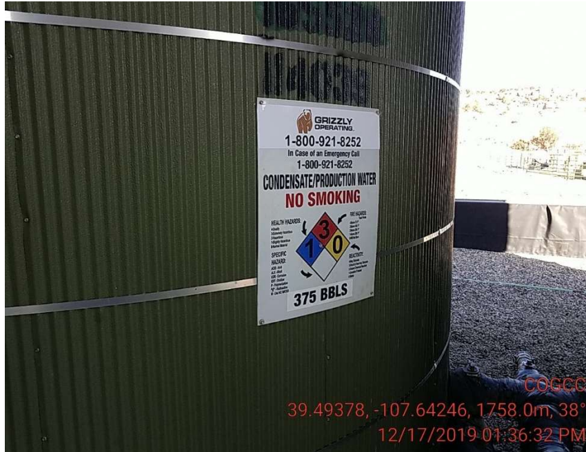
Sign is installed
